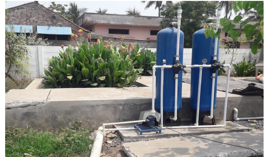
Phytorid Plant for treating Waste water
